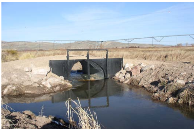
Emergency Watershed Protection Program (EWP) repaired two water control structures
